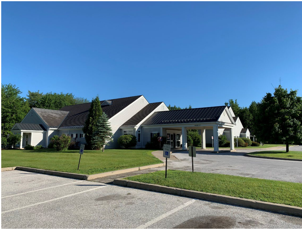
Community Health Center Rutland Region- Castleton
