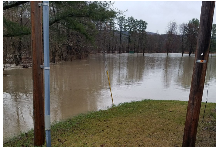
Inundation Flooding at North Road Well – April 2019
